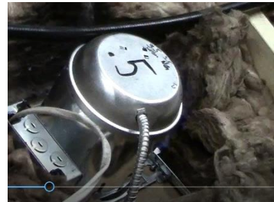
Figure 67 Test 5.5 escaping gas sustained burning on the inside of the recessed light's fixture's housing.
