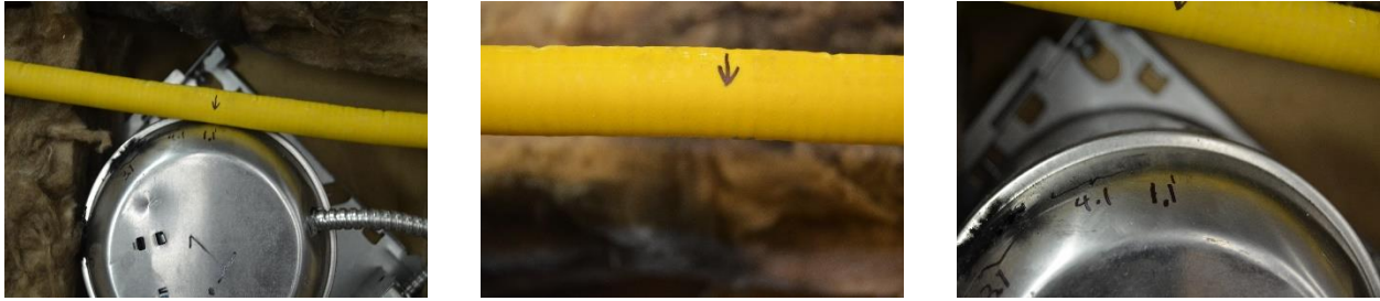
Figure 12 Test 1.1 in place (left). Undamaged WARDFlex® (center) and light fixture (right) post-test.
