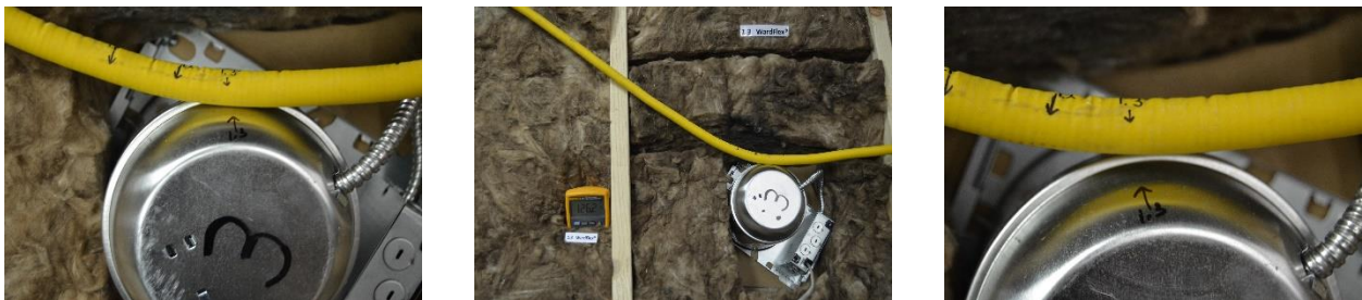
Figure 14 Test 1.3 in place (left & center). Undamaged WARDFlex® and light fixture (right) post-test.
