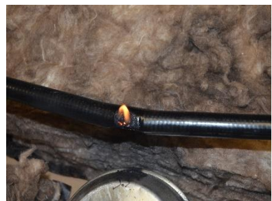
Figure 61 WARDFlex® Max outer jacket burning with gas turned off.
