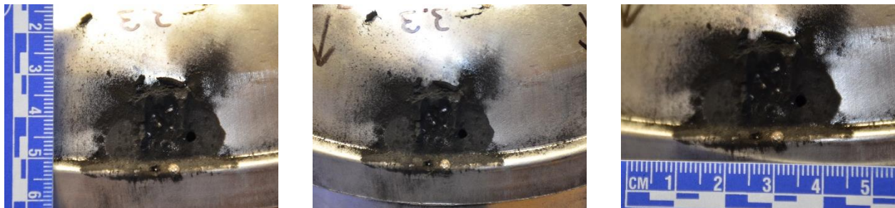
Figure 34 Damage to light fixture in test 3.3.
