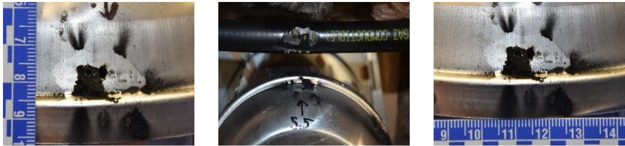
Figure 66 Damage to light fixture in test 5.5.
