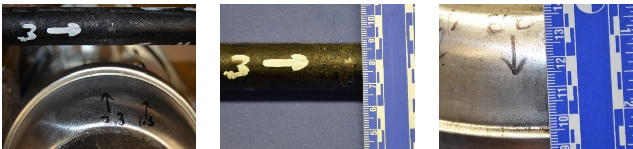
Figure 22 Test 2.3 post-test damage.
