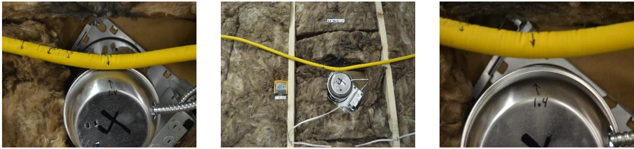
Figure 15 Test 1.4 in place (left & center). Undamaged WARDFlex® and light fixture (right) post-test.
