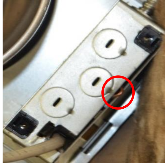
Figure 1 Electrical Short to Light Fixture Housing.
