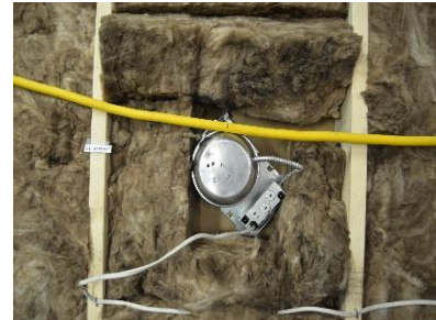
Figure 10 WARDFlex® in contact with recessed light.
