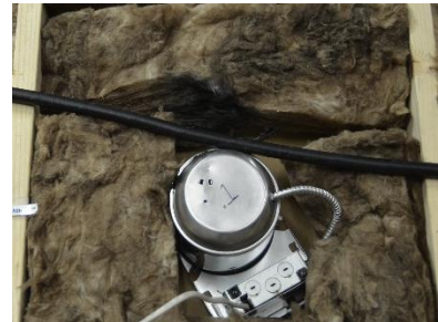
Figure 42 FlashShield™ CSST in contact with recessed light fixture.
